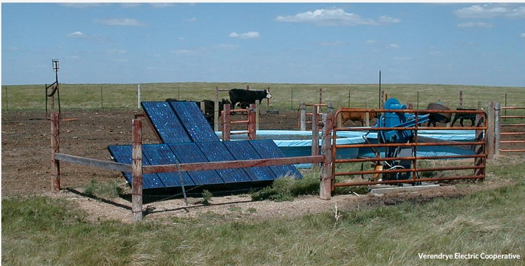
Solar-powered pumps for stock tanks.
