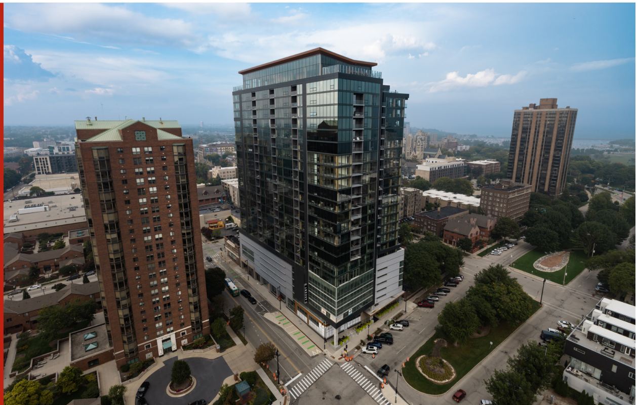
Completed in 2022, the Ascent MKE, a 25-story apartment building in Milwaukee, Wisconsin, is the world’s tallest building made from mass timber, a sustainable, fire-resistant wood construction material. “New apartments are the safest type of housing there is in the U.S.,” says Alex Horowitz, project director of Pew’s housing policy initiative.
