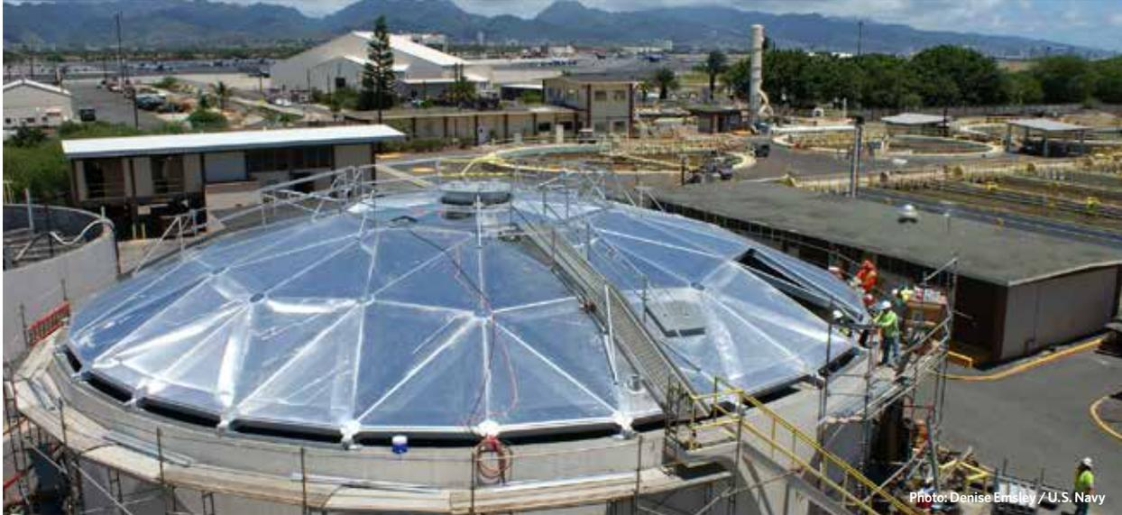
Naval facilities engineering teams upgrade the wastewater treatment plant at Joint Base Pearl Harbor-Hickam in Hawaii by replacing the floating steel roofs with fixed aluminum dome covers in 2011. The new covers help capture methane gas for future energy projects and for use as an alternative fuel source.
